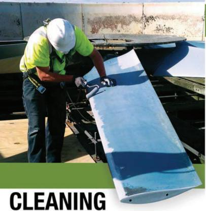
WITH OUR PATENT PENDING NEW PROCESS WE RESTORE COMPOSITE FAN BLADES FOR COOLING TOWERS TO 'NEW'.
